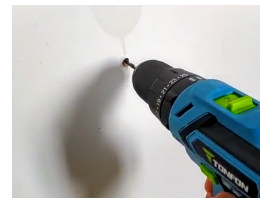
Figure 2: Drilling for sensor embedding.
